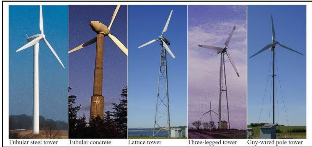
Fig 7.8: Wind Turbine Tower Design
